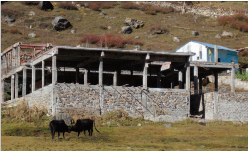
Construction of the ashram in Badrinath.
